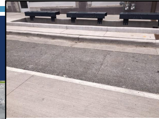
4-ft wide Porous Pavement Roadway
